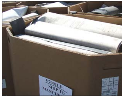
Worker from D7 Roofing Services collects older roof membrane prior to installation of new EnergySmart Roof system atop the Burlington Coat Factory retail store. The older membrane is packed into boxes and shipped to Sika Sarnafil for recycling.
