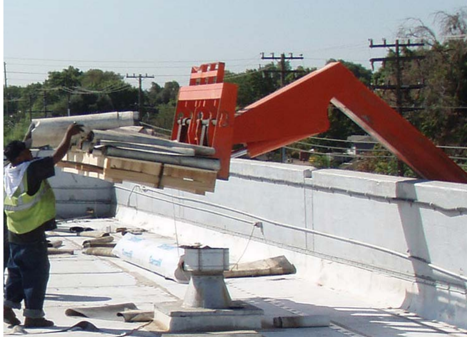
Worker from D7 Roofing Services collects older roof membrane prior to installation of new EnergySmart Roof system atop the Burlington Coat Factory retail store. The older membrane is packed into boxes and shipped to Sika Sarnafil for recycling.
