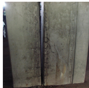
Column Deflection at Expansion Joint
