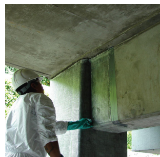
Installation of Glass FRP
