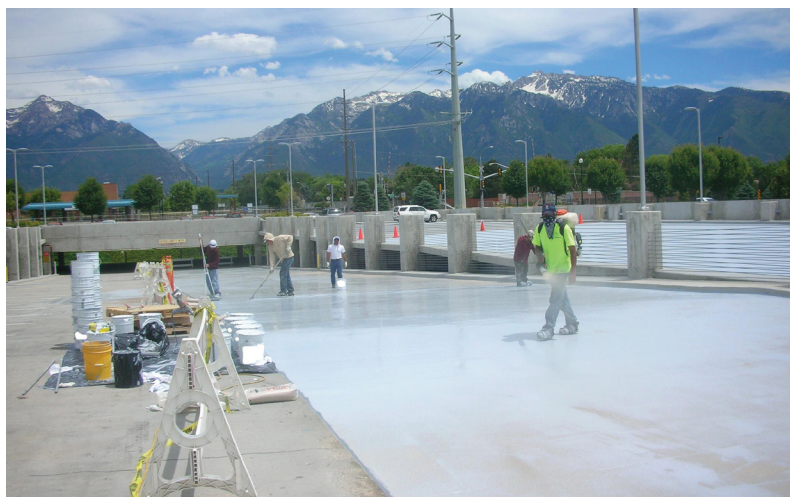
Elastomeric Membrane Top Coat Application with Aggregate
